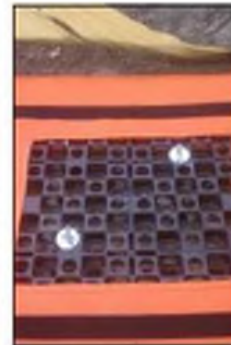
Install base with 2 to 4 anchors as needed.
