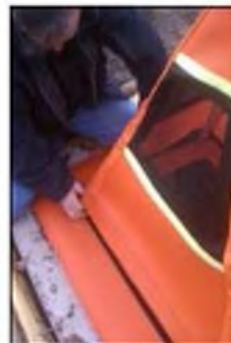
Tightly secure base to tower.
