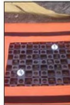
Install base with 2 to 4 anchors as needed.
