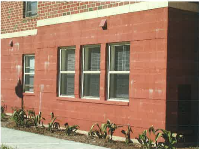
Fig. Efflorescence at CMU wall at Spartan Suites.
