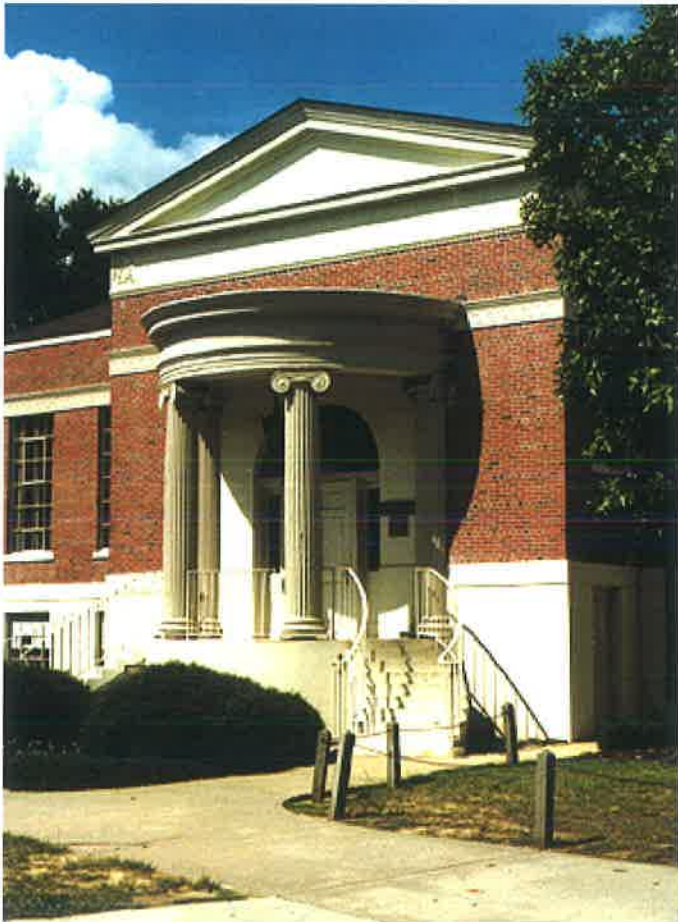
Fig. Primary entrances should have a canopy. This feature can be expressed in a variety of styles, modern in the top image or classical as seen in the bottom image.
