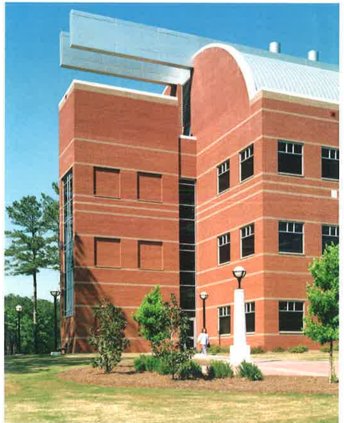
Fig. In the image above, the rhythm of the fenestration has been continued onto a wall that would otherwise be a large field of undifferentiated brick by establishing the location of false window openings and then infilling them with brick.
