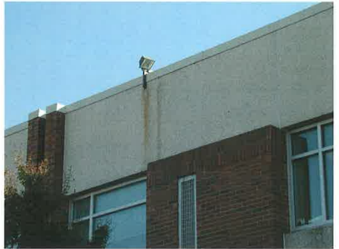
Fig. Improvised site lighting and drainage issues.
