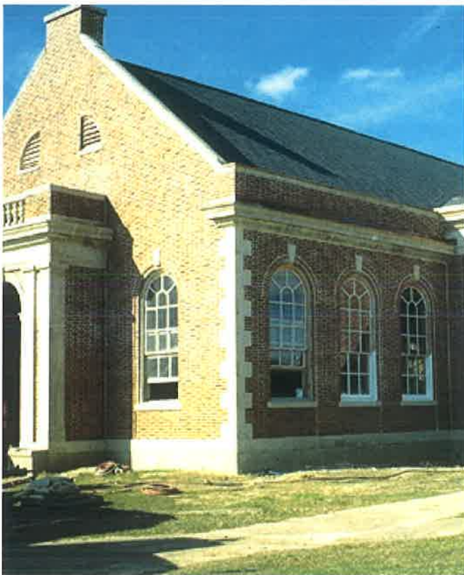
Fig. Stone accents may be used at a variety of locations. Keystones above windows, lintels, pediments, corner supports and base materials provide texture and augment the overall aesthetic quality of buildings. These accents may be classical or contemporary in style.
