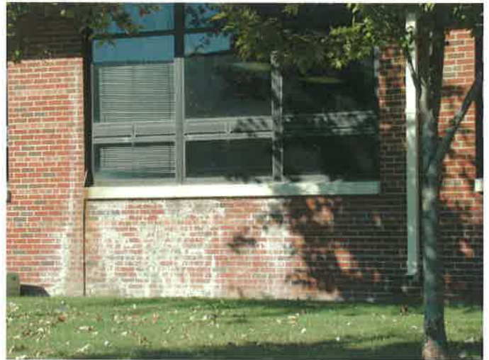
Fig. Water penetration at Brown Hall.
