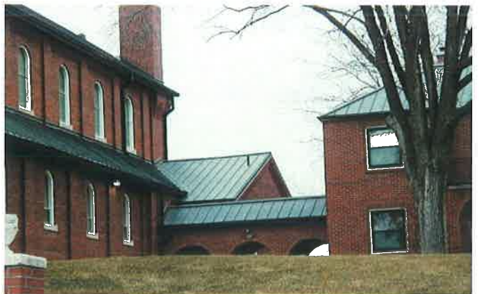
Fig. In both cases, the roofing material is a metal standing seam with a grey finish. In the top image the roof pitch is 4:12 and the bottom image is 12:12.
